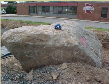
This 20 cubic yard boulder held up construction
